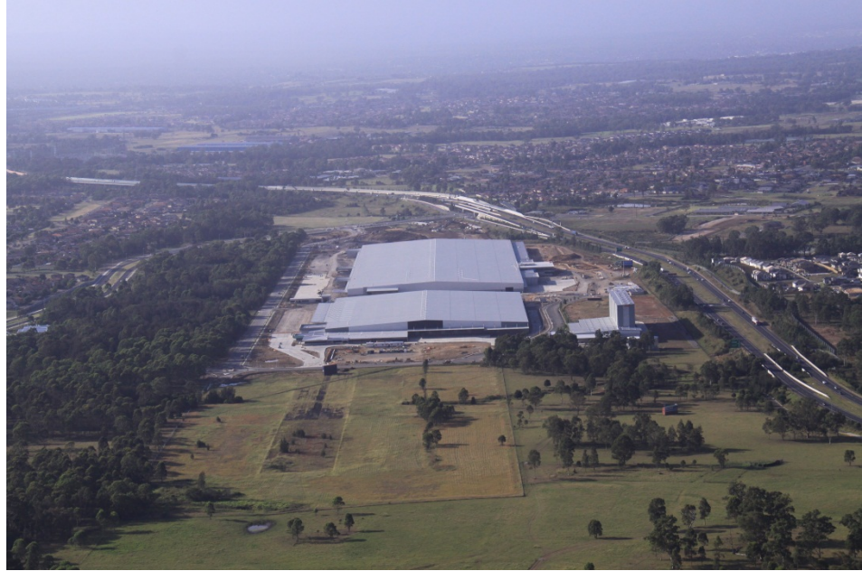
Figure 2 – Elizabeth Hills in the foreground and warehouse buildings being constructed as viewed looking towards the south
